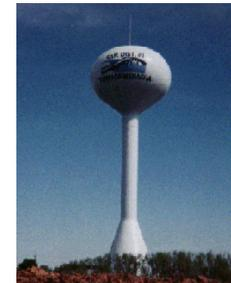
The West Side System consist of four wells, two treatment plants, two one million gallon reservoirs, and two 300,000 gallon water towers.
